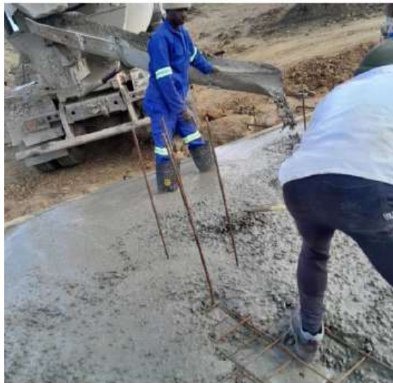
Pouring of concrete for causeway
