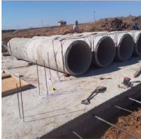
Preparation for a top slab- causeway
